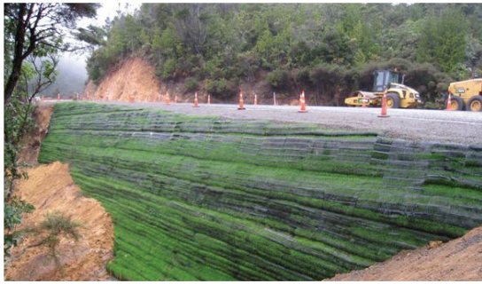
300mm Siltstop used for road support (State Highway 26, New Zealand).
