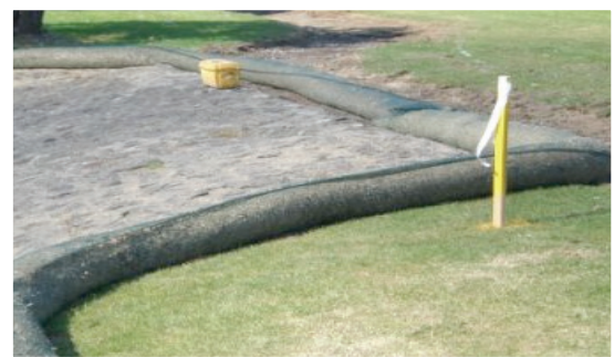
300mm Siltstop used as cost-effective silt fencing for construction projects (Manukau, NZ)
