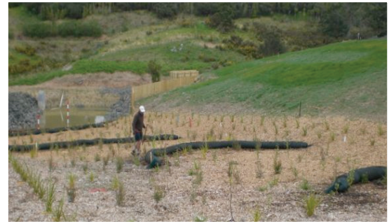
300mm Siltstop used to control overland flow velocity thereby removing sediment and other debris by sedimentation and filtration
